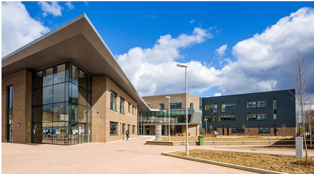
Figure 4 – Morriston Comprehensive (BREEAM Excellent) 2
